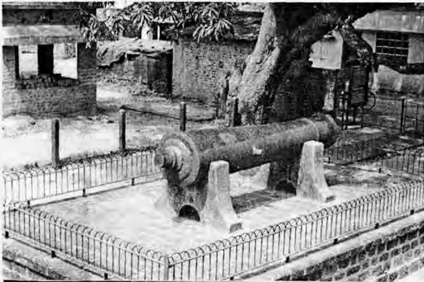
Fig. 1: The forge welded iron cannon at Bishnupur.
